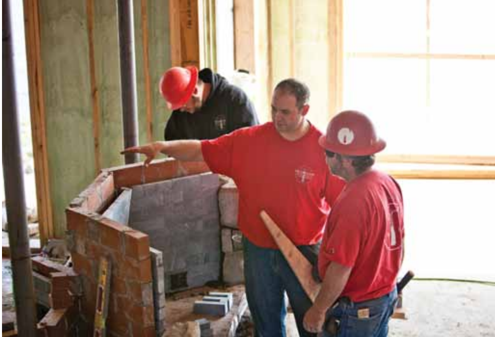
George Libby Sr., Mike, and George Jr. (opening spread) stand before a retaining wall of old New England wall stone that they're constructing at a Muscongus Bay home. The veneer on the detached garage (above, left) matches the wall. A two-and-a-half story granite fireplace with a soapstone brick interior will define the home's great room (above, right). A masonry hammer (opposite, top), which has a chisel on one end, is used to shape the stone. When a worker, pictured with the retaining wall (opposite, bottom), needs to make a large cut, he employs a diamond saw.
